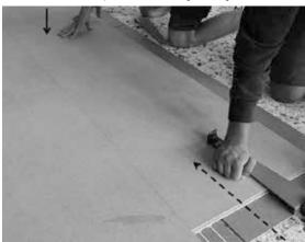
Place the pull bar support against the edge of the lower board so as not to damage the connection system. For a perfect panels fitting, it be may helpful to apply a load located near to the junction of the 2 panels previously installed.
