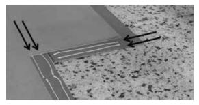
2. Hold the panel to be connected at 45  $^{\rm o}$  and fit it into the <code> wfold/down</code> click system.
