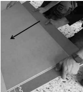
For a perfect panels fitting, it be may helpful to apply a load located near to the junction of the 2 panels of the previous line..
