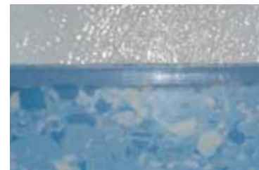
HOT-WELDED DECOCHOC Panel / panel or panel / floor hot-welding
