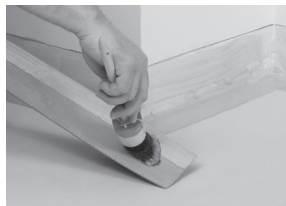
Apply glue on the floor and against the wall till the line.
