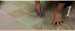
Put a non-migrating double-sided adhesive or bonding tape under the seal before double cutting.
