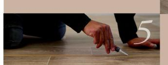
Insert the end of the nozzle in the joint and work backwards, slowly injecting the fluid until it overflows at the surface on the paper adhesive tape.
