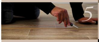
Remove the masking tape and clean off any remaining traces of welding fluid using white spirit. Avoid walking on the joint for 24 hours. Insert the end of the nozzle in the joint and work backwards, slowly injecting the fluid until it overflows at the surface on the paper adhesive tape. Leave the welding fluid to act for more than 1 minute.
