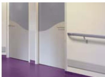
WALL PROTECTIONS & HANDRAILS
