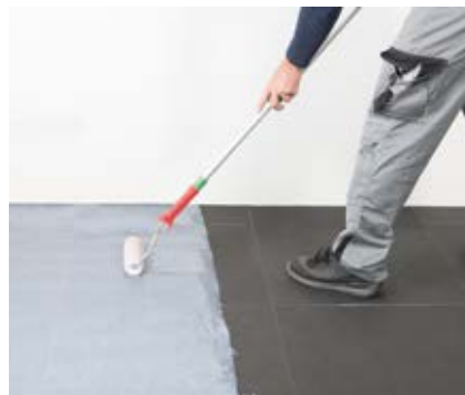
Application of the pressure sensitive adhesive
