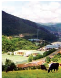
Gerflor Tarare manufacturing plant
